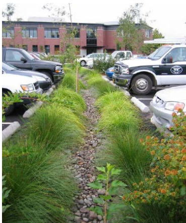
Figure 4 Example of Vegetated swale to promote infiltration. (EPA 2015)
