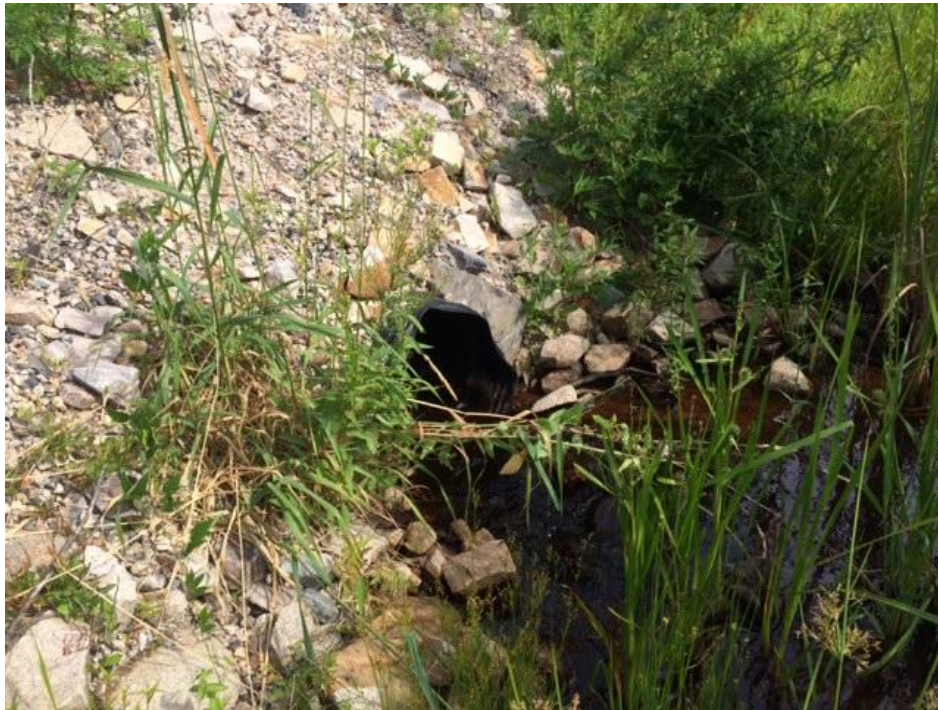
Looking east, close-up of 15" culvert inlet – Area L
