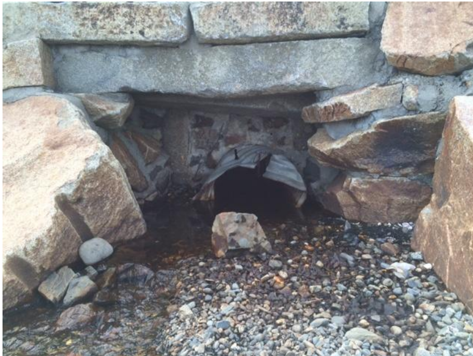
Close up of 24" culvert outfall – Outfall Area L
