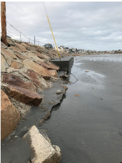
Photo 3: Undermining of existing seawall.
