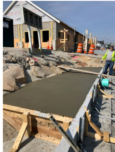
Photo 10: Pouring of concrete step.
