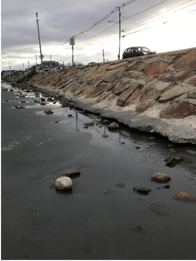
Photo 1: Undermining of existing seawall.
