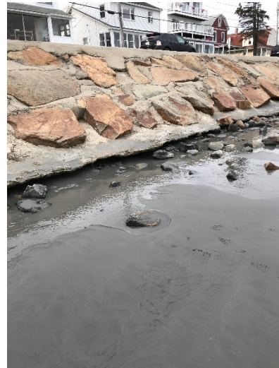
Photo 2: Undermining of existing seawall.
