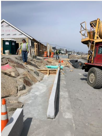
Photo 9: Placement of vertical granite step.
