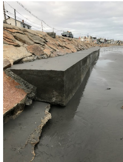
Photo 4: Undermining of existing seawall.
