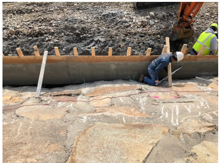
Photo 6: Forming for 4 th pour north of Bathhouse.
