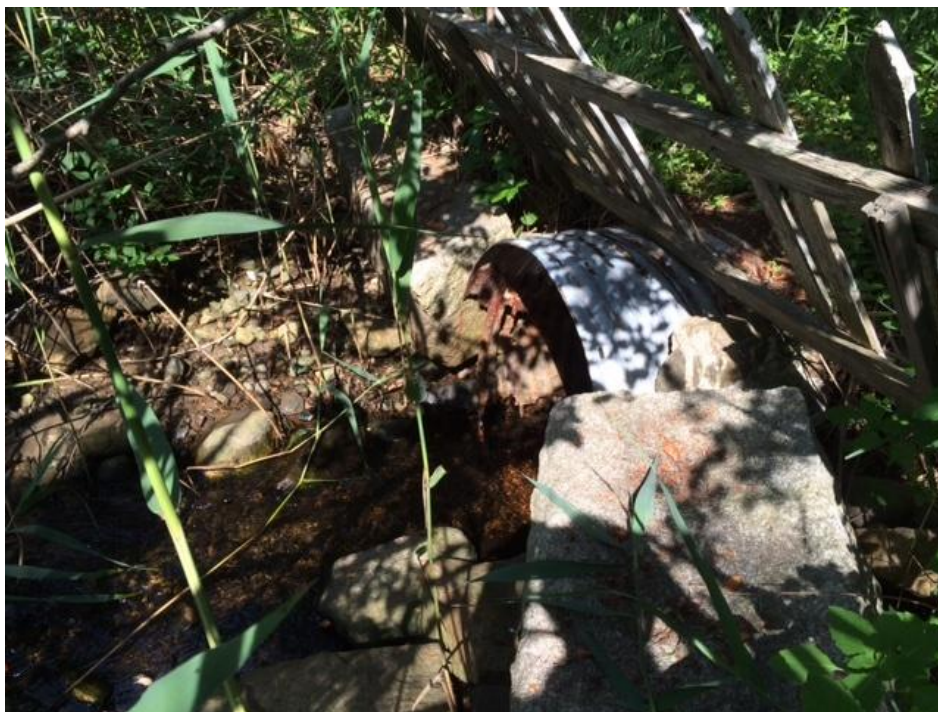
Looking north, close up of 36" culvert inlet – Area J
