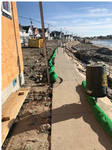
Photo 11: Newly placed erosion control sock as requested by the DEP.
