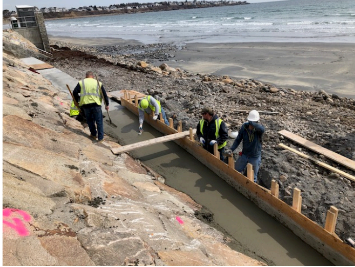
Photo 7: Forming for 4 th pour north of Bathhouse.
